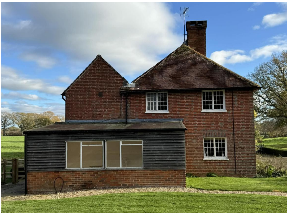
Fig 3: The west elevation showing a single storey side extension added in the late 20 th Century. A first floor extension was added with a gable end to the rear of the building (left side).
