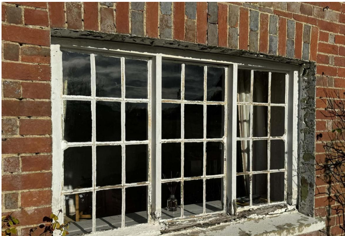
Fig 5: An example of an existing late 19 th Century window from the principal elevation. They sit inside of plainly finished timber frames with metal glazing bars sat inside, also found on each side of the dwelling.
