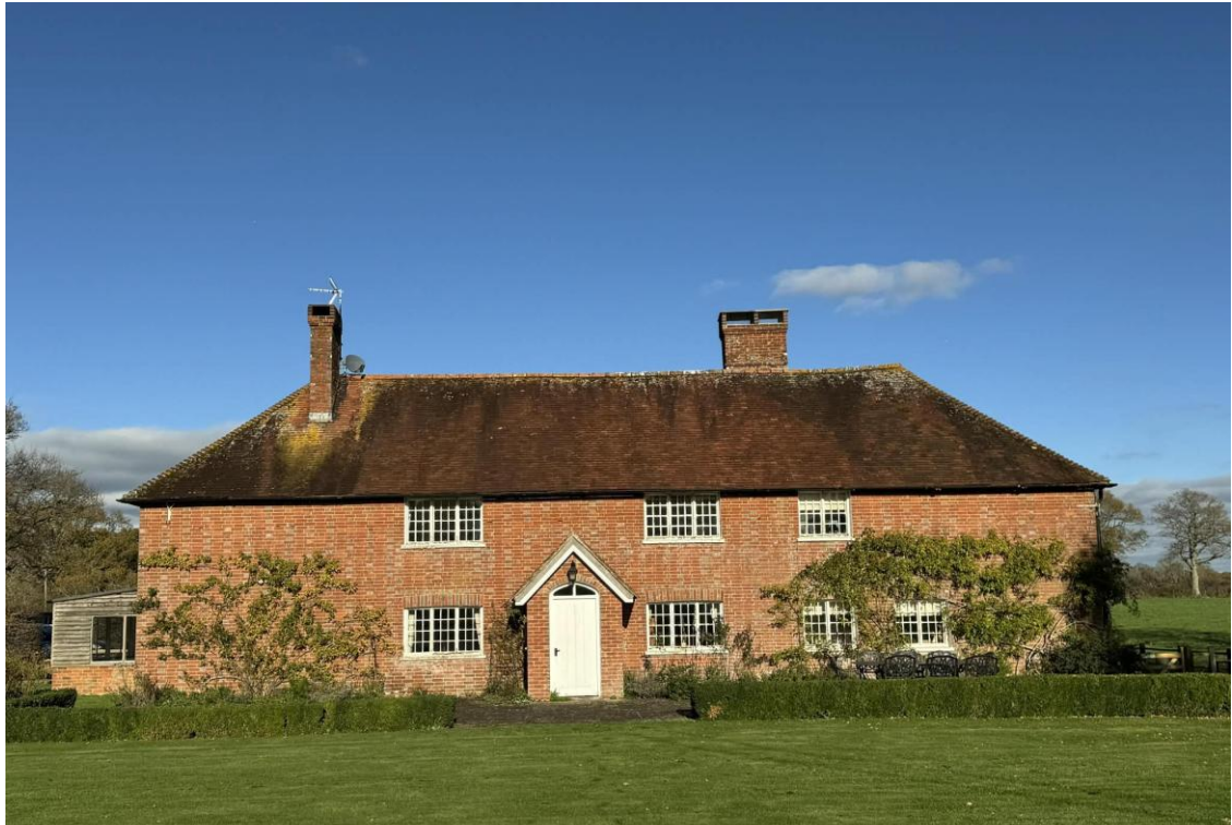
Fig 2: Jendens Farm dates from the 17 th Century if not earlier and was refaced in brick in the early 19 th Century. Its principal elevation as shown here faces south, from where the heritage asset is best appreciated.
