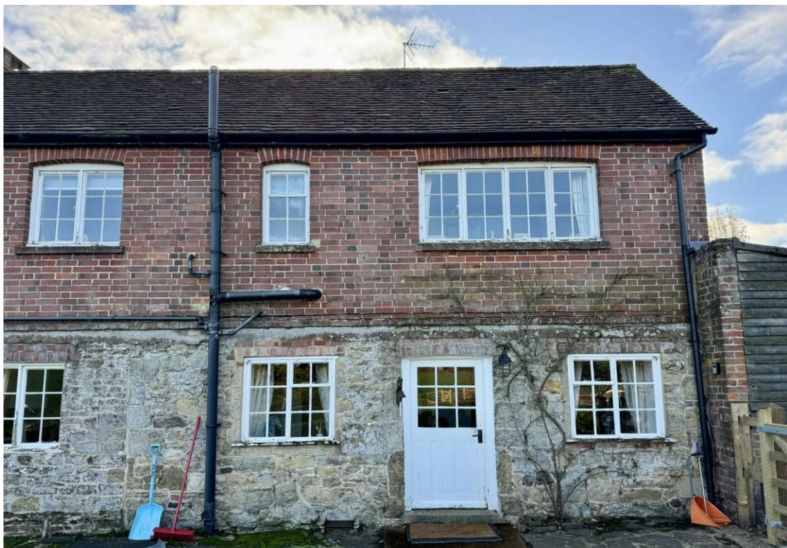
Fig 7: This rear facing elevation contains modern Crittall windows added when the building was extended.
