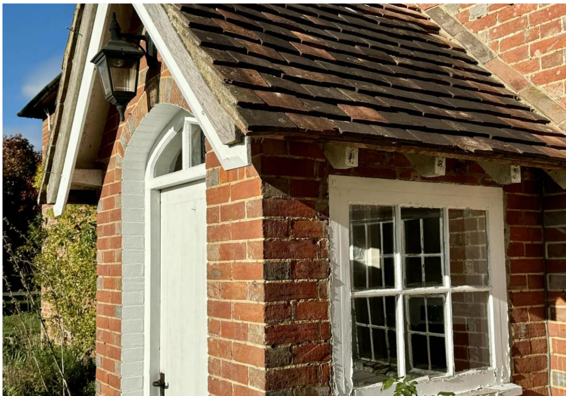
Fig 9: The windows to each side of the porch are believed to be the oldest and considered historic fabric.
