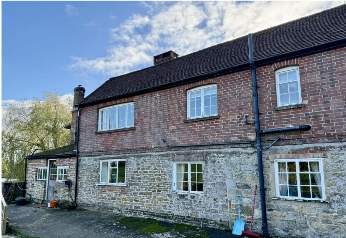
Fig 6: At the rear to the north side, a single storey stone wall comprises what was once a single storey lean-to, like that to the left with the door, which was extended in the late 20 th Century with a first floor brick extension.
