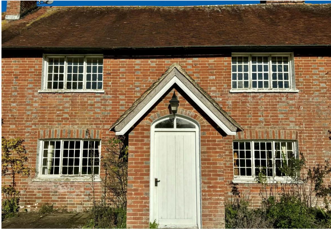
Fig 4: Jendens Farm is a Grade II listed building and is of a timber frame construction. Metal casement windows were added to the front and sides in the late 19 th Century, replacing earlier sash style casements.
