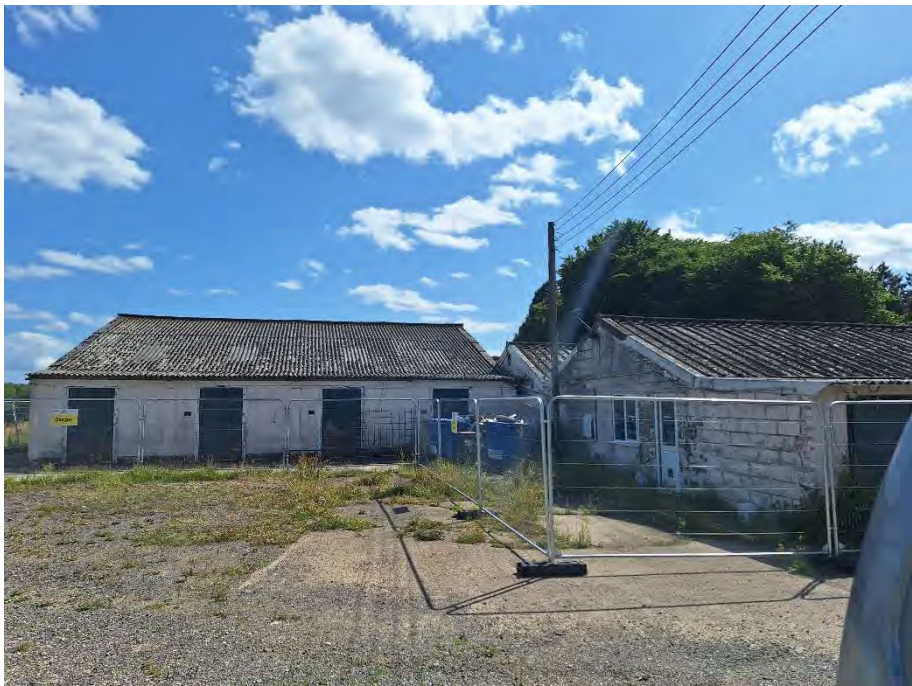
Plate 1: Existing central farmyard buildings looking south.
