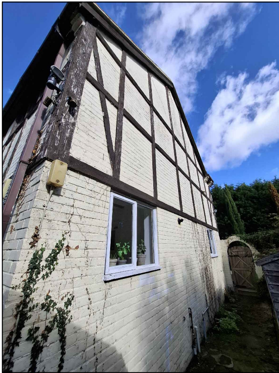
EXISTING SIDE VIEW (6)
