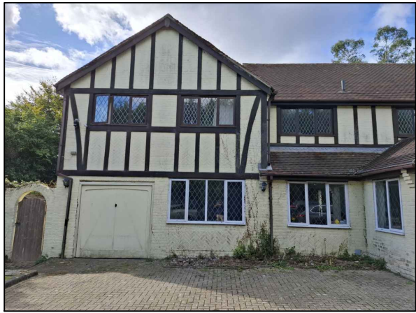
EXISTING VIEW TOWARDS GARAGE (1)
