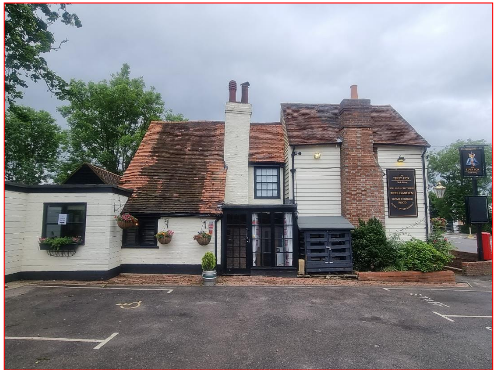
Plate 4 View of south elevation to the Topsy Fox Public House, taken from the car park.
