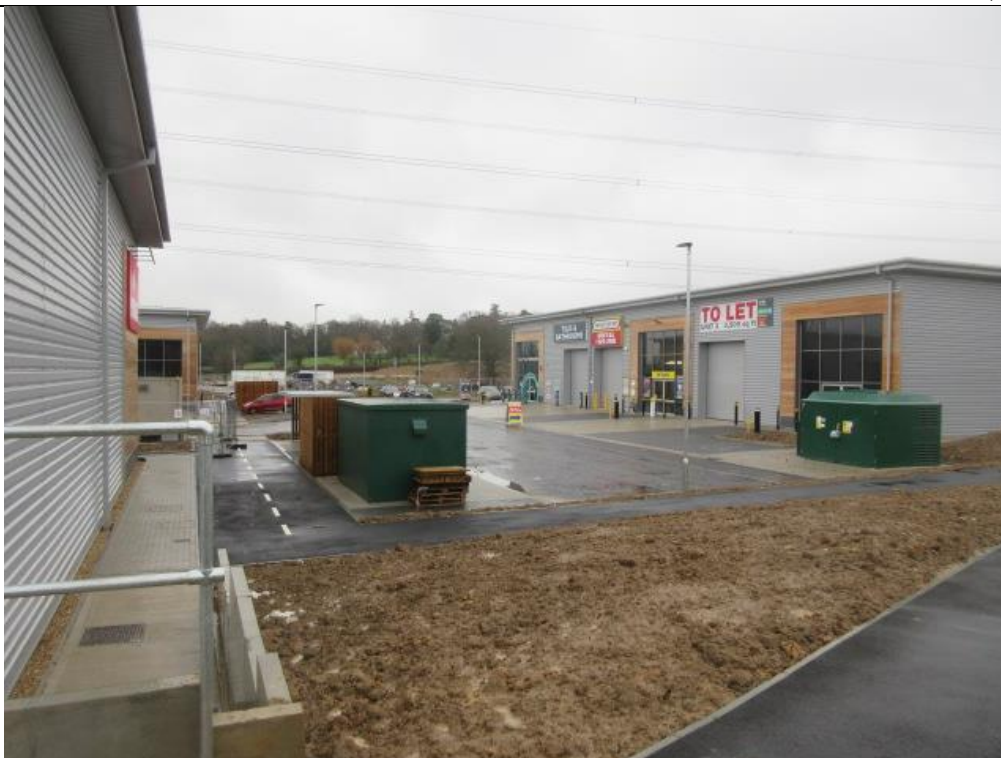
Plate 3: New commercial development north-west of the site
