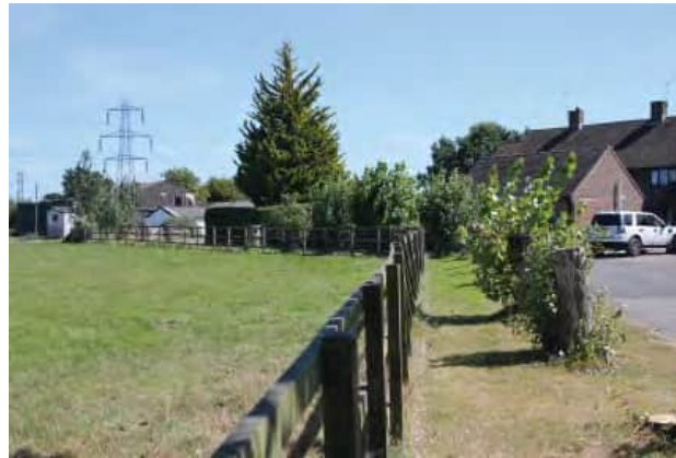
Post & rail fencing along southern boundary with Hilland Farm Cottages
