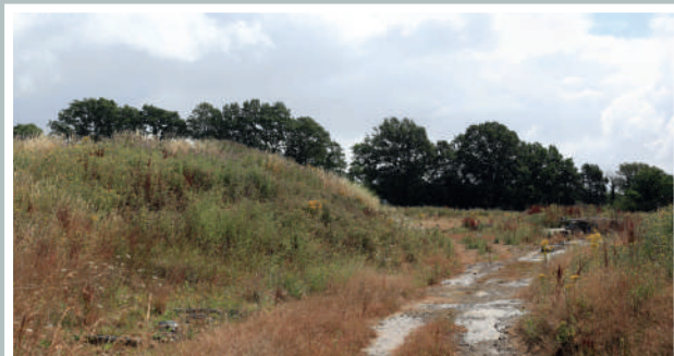
Photo J- Bunding at the site entrance
