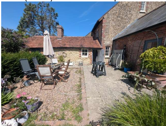
Rear (south) elevation and patio
