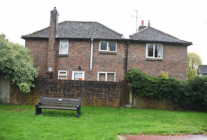
Side (north) of building: Note this is all extension so all windows here to be replaced.
