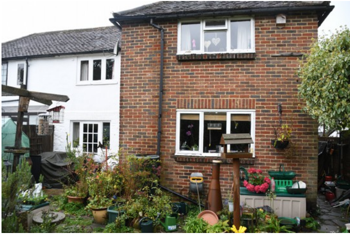
Rear (east) of building: Original building windows (to the left in the photo) to be retained. ONLY extension windows to be replaced.
