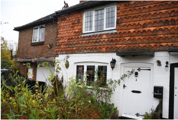
Front (west) of building: Original building windows (to the right in the photo) to be retained. ONLY extension windows to be replaced.
