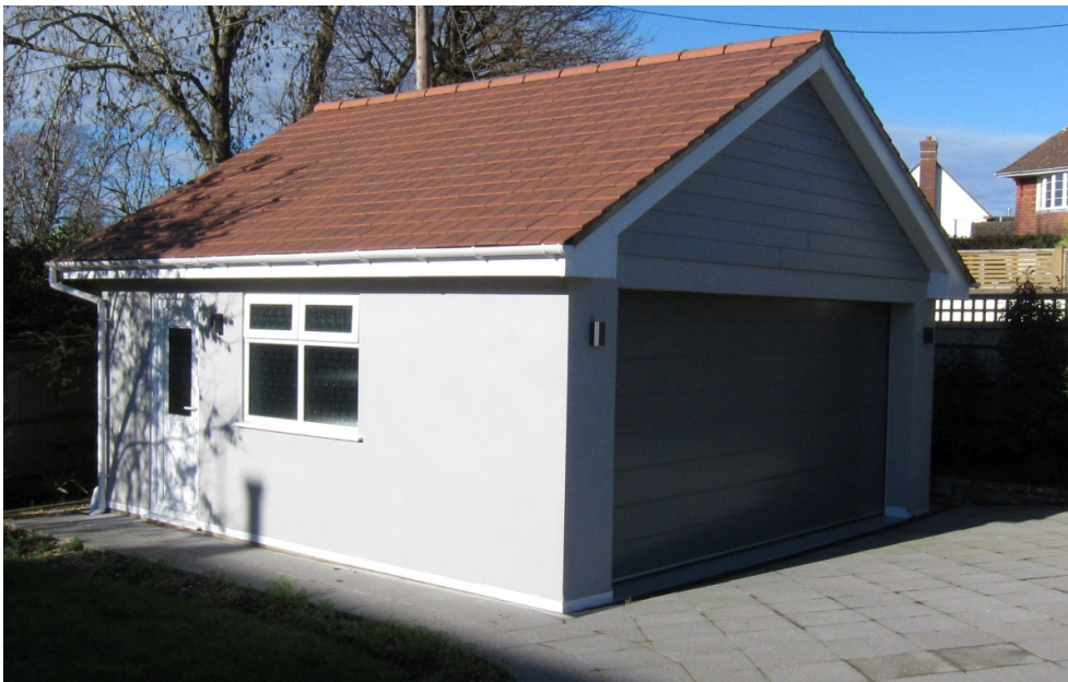
New detached garage built under planning approval DC/21/1123
