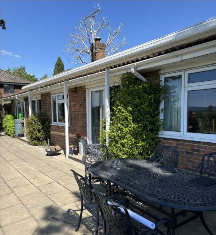
View towards the rear of the dwelling from the garden terrace
