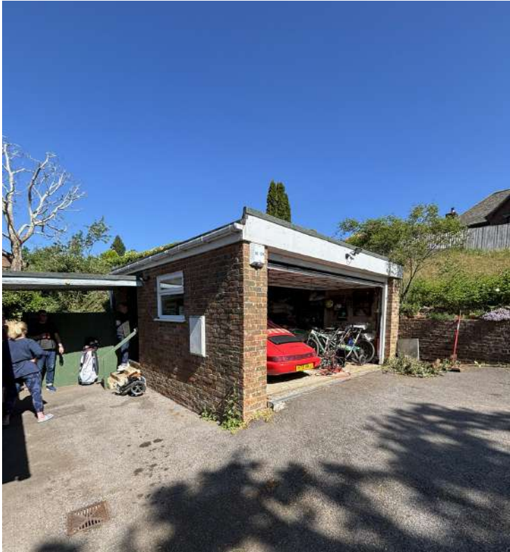
View towards the covered external link between the dwelling and garage
