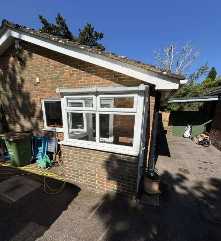
View of the existing side / ancillary entrance into the Kitchen
