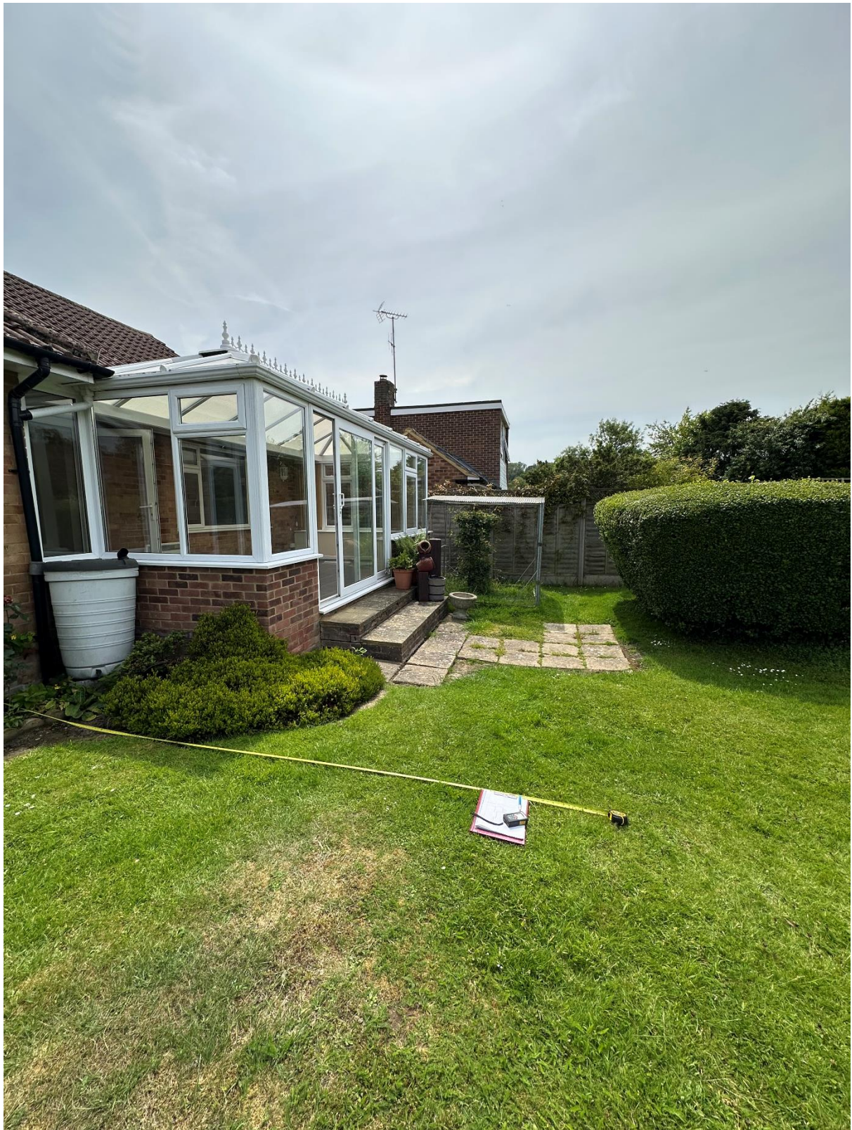
Image shows the rear elevation, conservatory and relationship with neighbour at 56, as well as a tape at 4.00M out from current wall.
