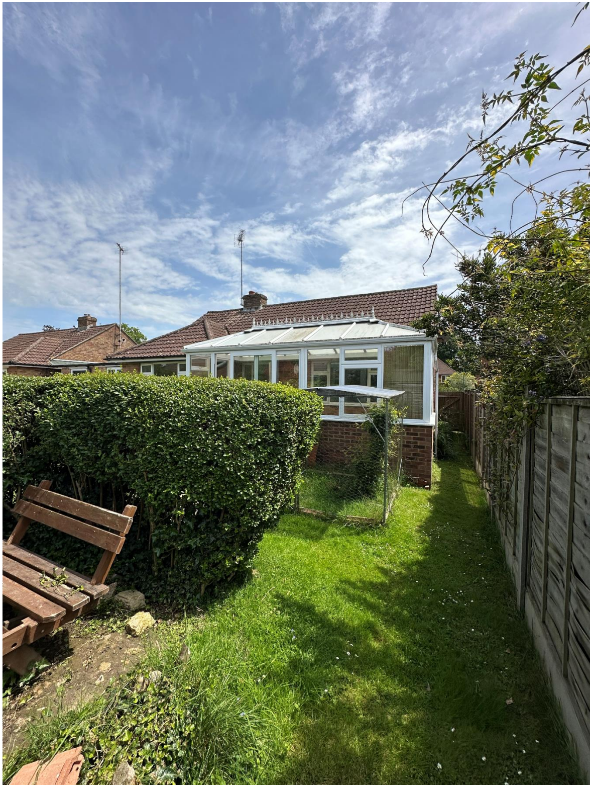
Image shows the rear elevation of the bungalow and side passageway with neighbour at 56
