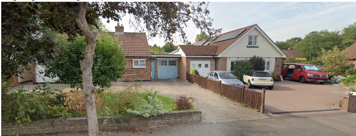
Image September 2020 – Post Nr 40 garage works
