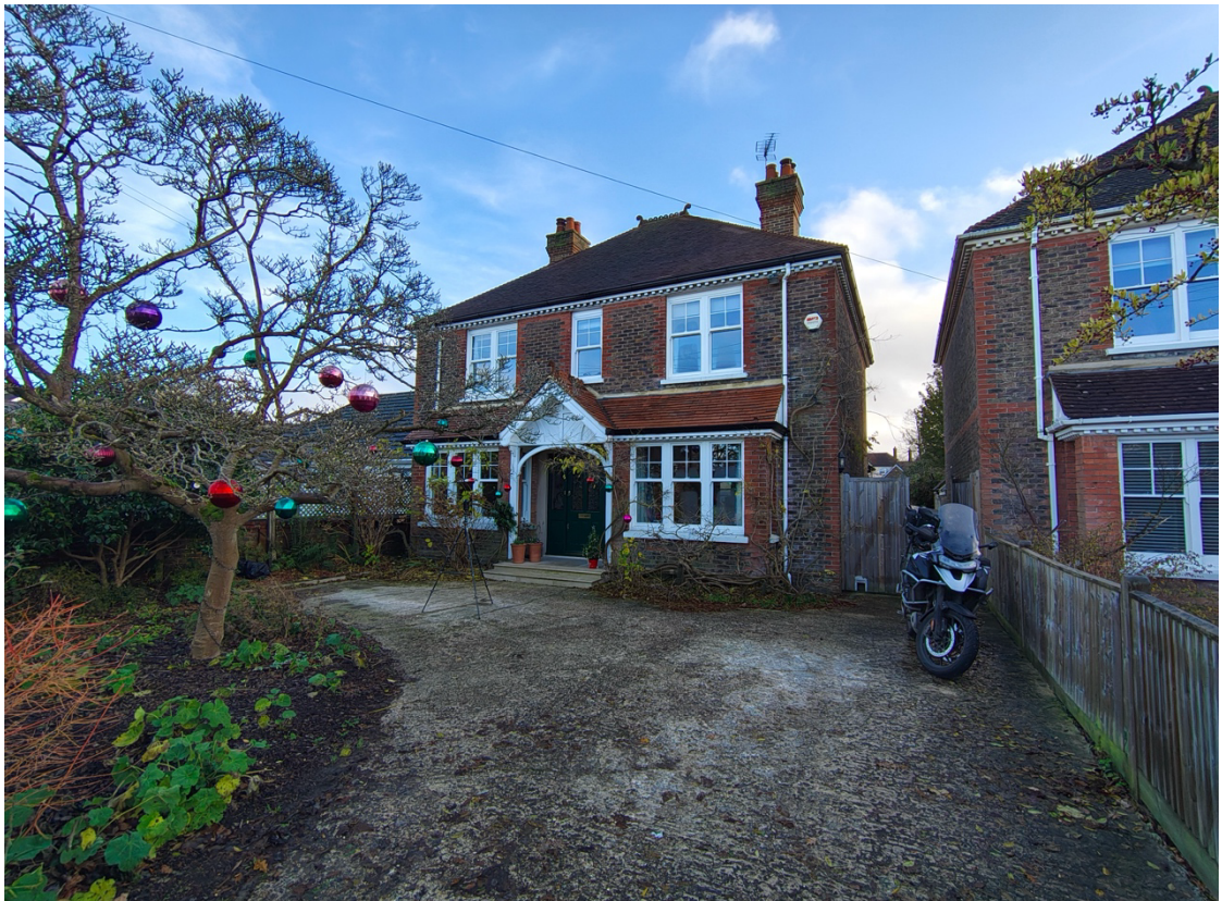
Figure 1. Photograph of the front of 34 Rusper Road
