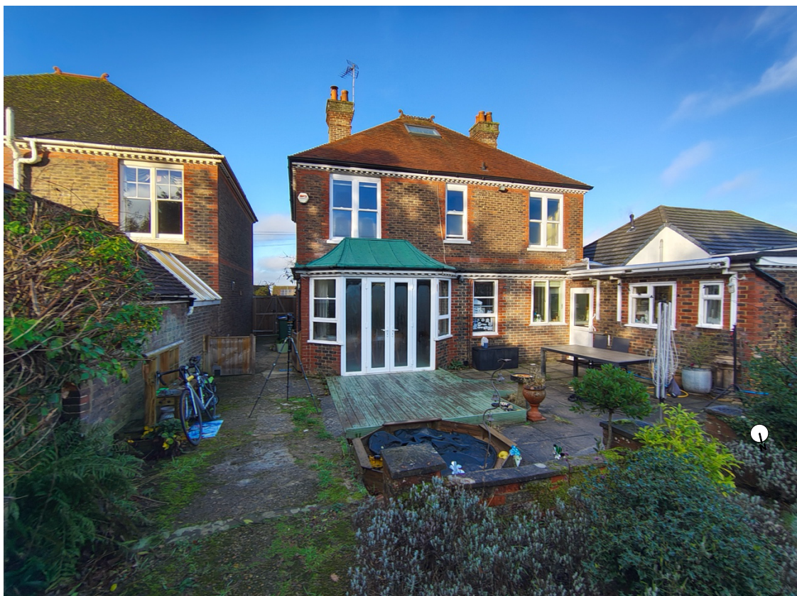
Figure 2. Photograph of the rear of 34 Rusper Road
