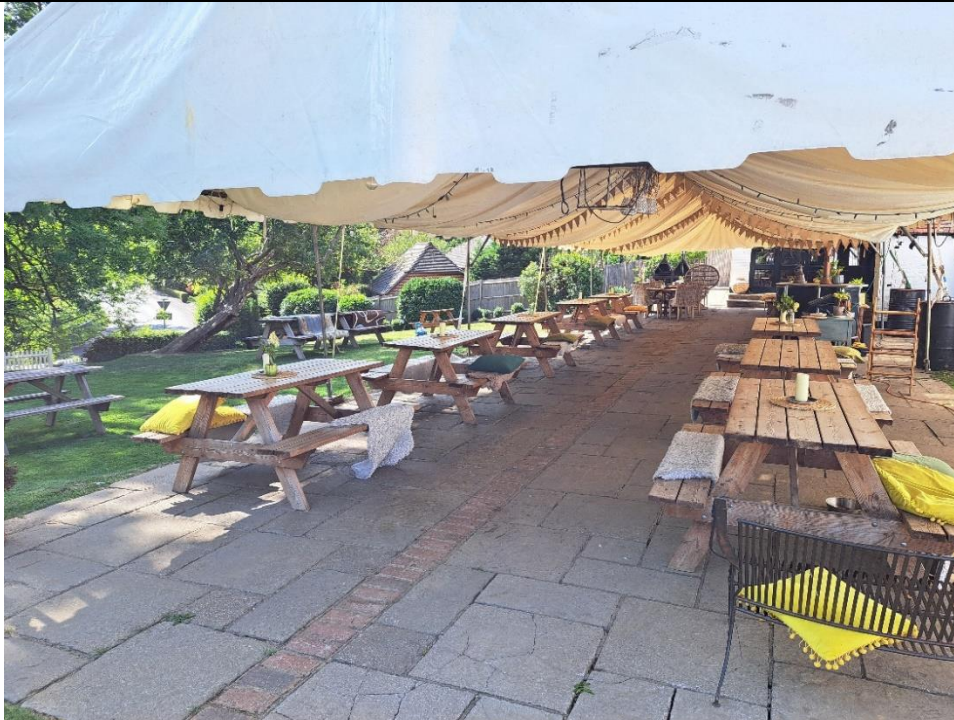
Area of hard standing forming paved patio to south of pub building/Site.
