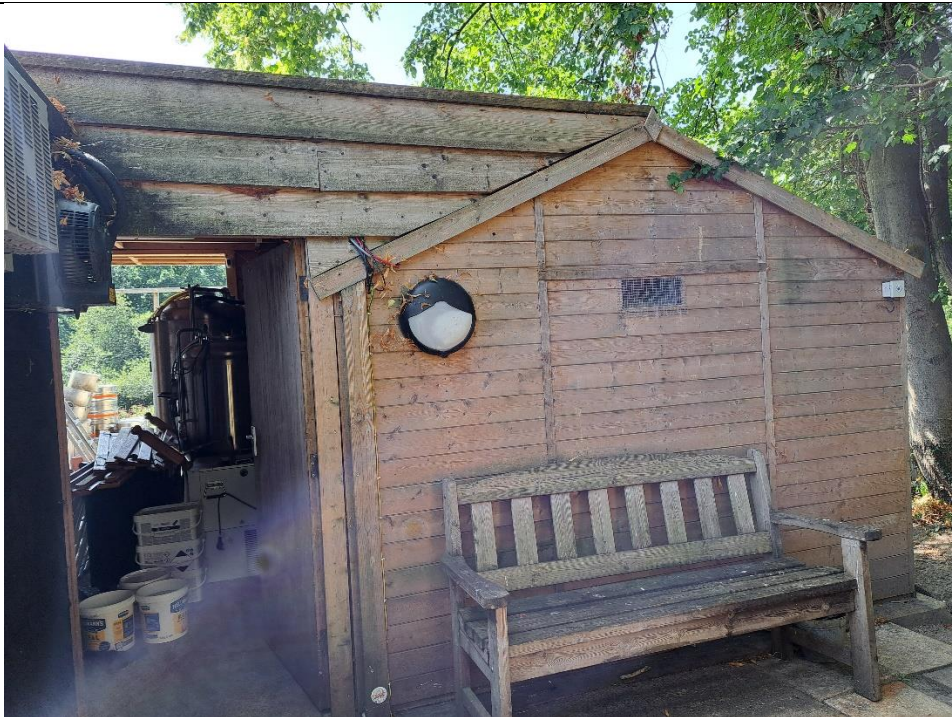
View of timber shed and canopy – North-east elevation.
