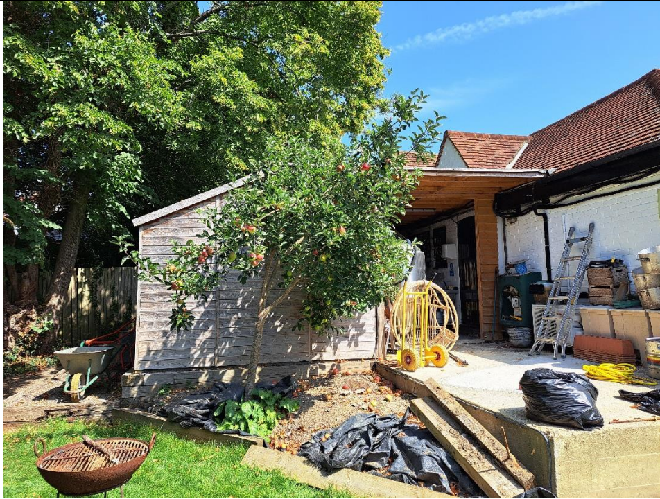
View of timber shed and canopy – South-west elevation.
