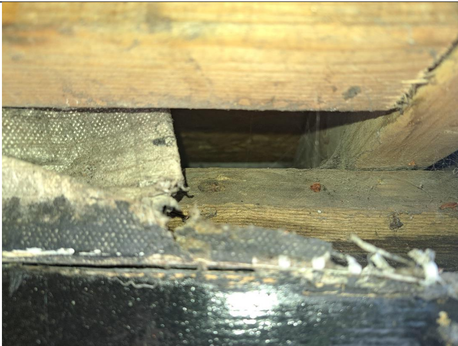
Close-up view of feature to right in photo 15 above.
