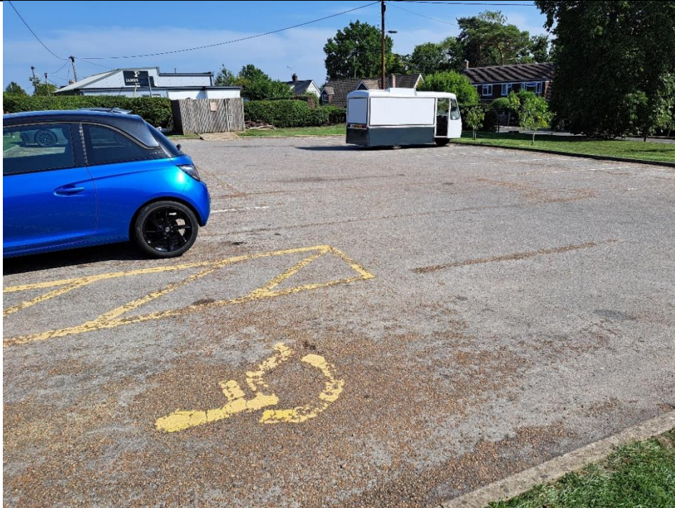
Area of hard standing forming car park to east of Site.
