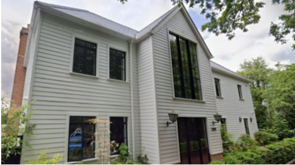
Figure 4.5 – Recently constructed dwelling on Mayes Lane
