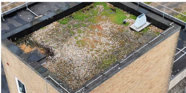
Plate 3.2 Shingle/substrate on the lift shaft roof on the east of the former Novartis building
