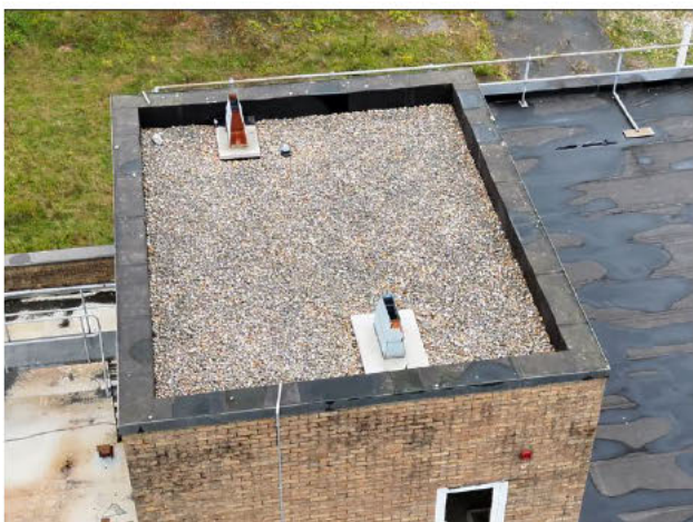
Plate 3.2 Shingle/substrate on the lift shaft roof on the east of the former Novartis building
