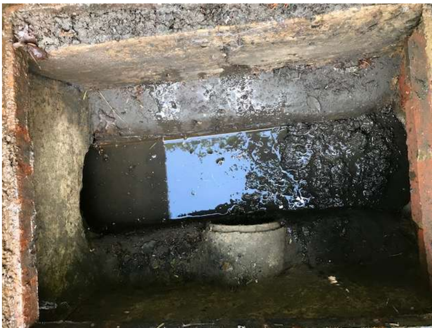
Silted up pipe on the left-hand side pipe immediately before and after blockages.
