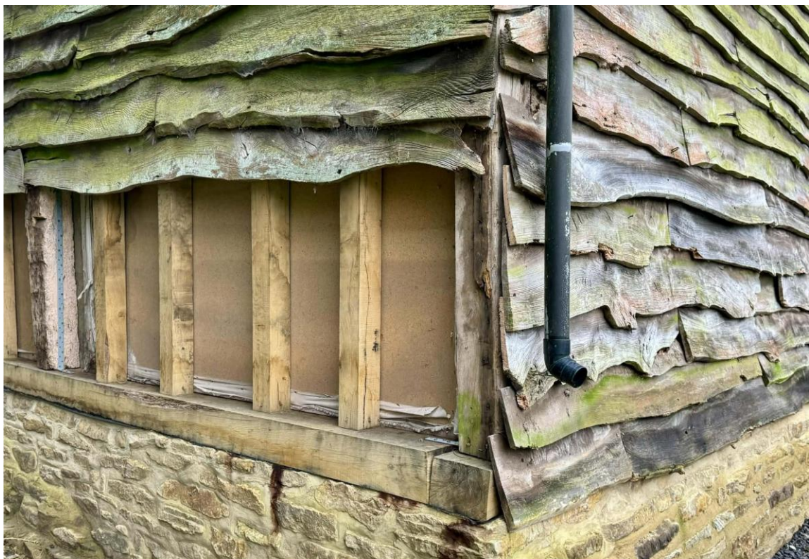
Fig 6: The former tithe barn dates from the 17 th Century and is timber framed on a stone rubble base.
