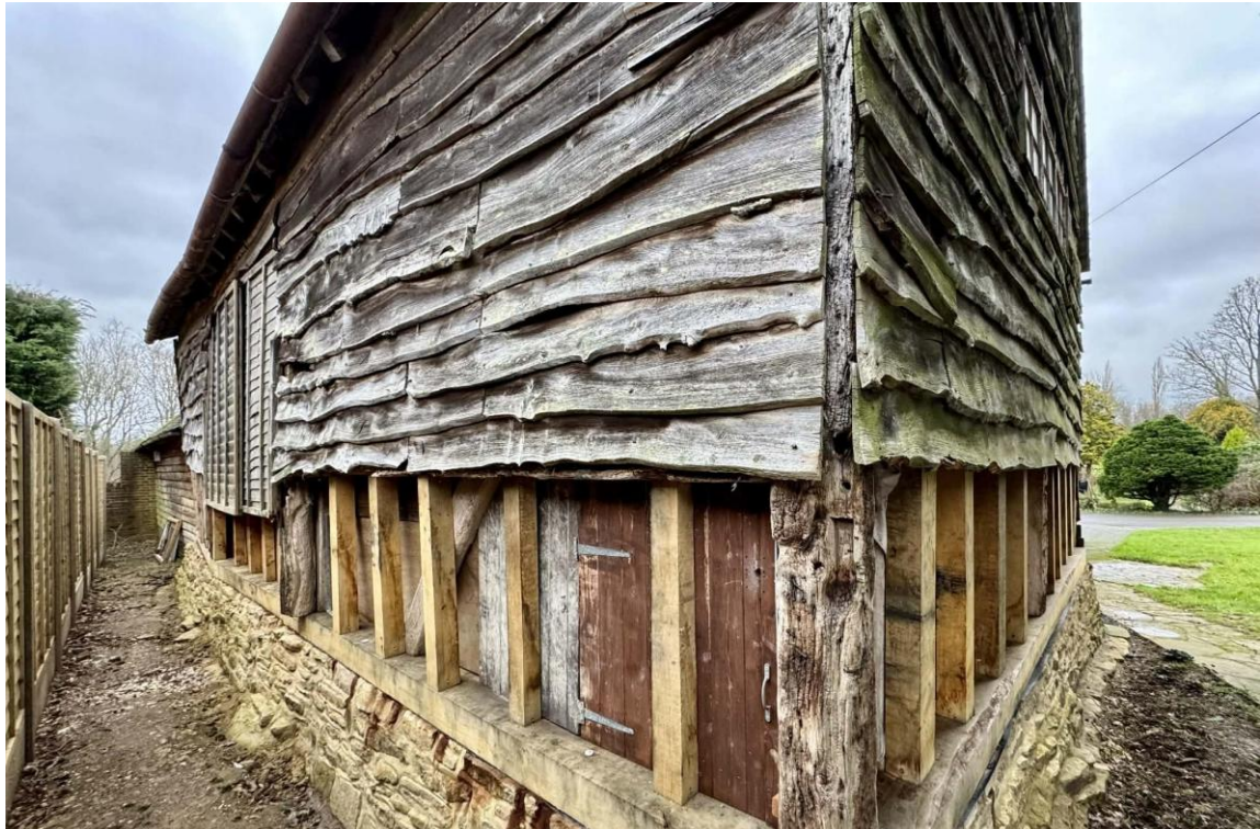
Fig 5: The historic tithe barn would continue to be used for ancillary use and repaired using traditional feather edged timber weather boarding, to uphold and better sustain the significance of the heritage asset.
