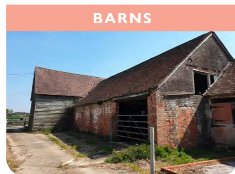
Existing historic barn
