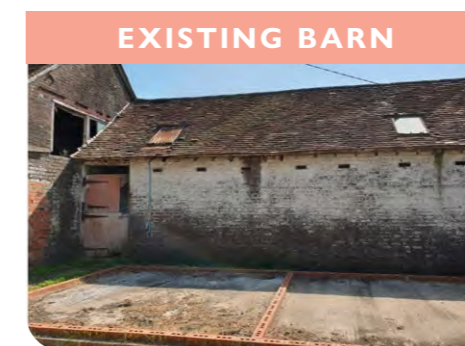
Existing late nineteenth century barn to be potentially refurbished
