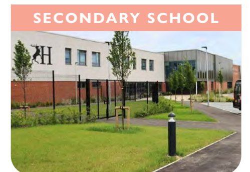
Bohunt School, North Horsham (Mowbray development)
