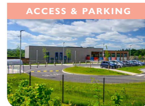
A clear access point with parking (Berkeley - St Peters Primary School)
