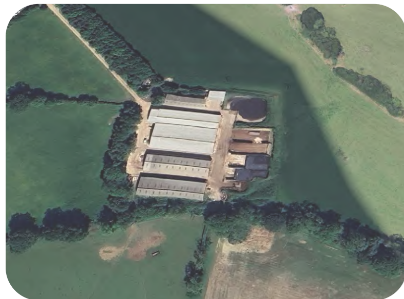
Sluetts Farm (Old dairy farm) to be demolished
