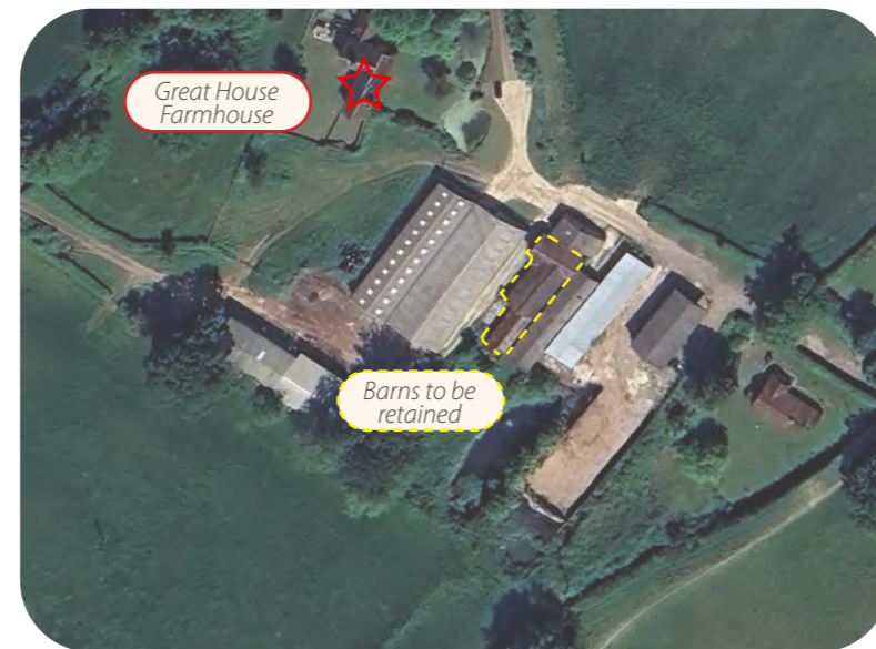
Historic Barns to be retained and surrounding later era structures to be demolished
