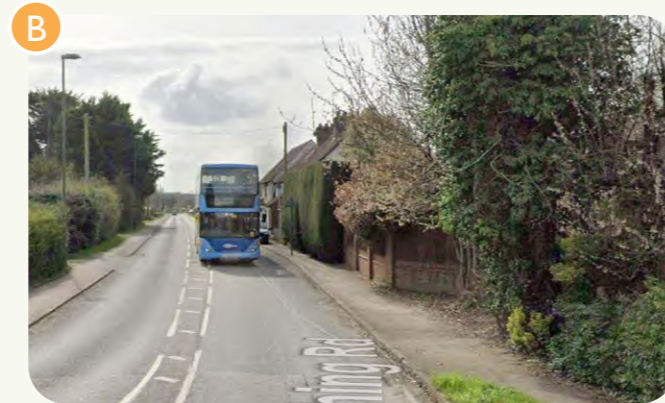
Bus stop on Worthing Road
