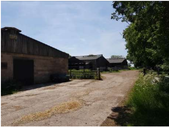
Photo 2: Western elevation of B2 in forefront, with western elevations of B3 and B4 in rear of photo.
