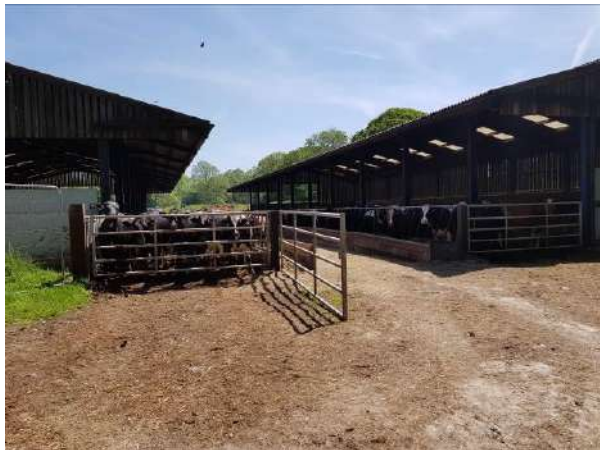
Photo 3: Southern elevation of B3 and northern elevation of B4.
