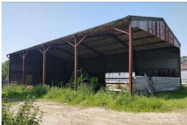
Photo 8: Northern and eastern elevations of B8.
