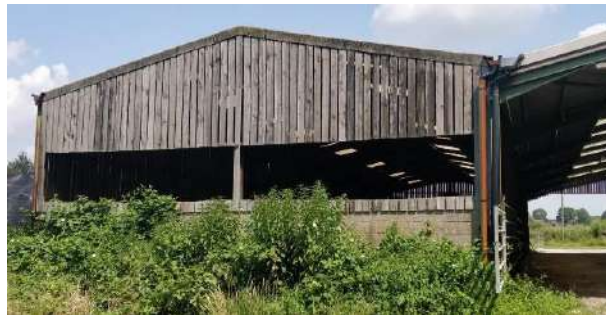
Photo 19: Southern elevation of western section of B15.
