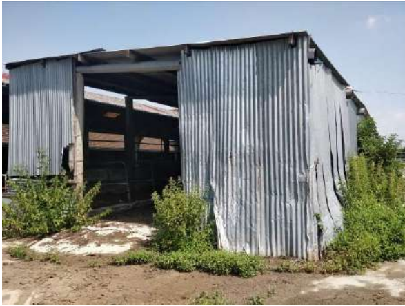
Photo 9: Southern and eastern elevations of B9.
