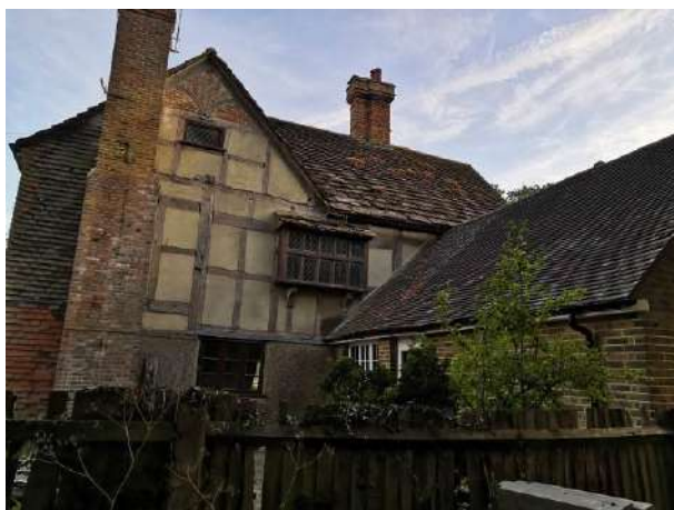
Photo 21: Northern elevation of B16.
