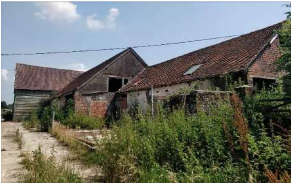
Photo 13: Western and southern elevations of B12.
