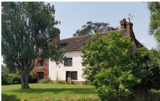
Photo 20: Eastern elevation of B16.
