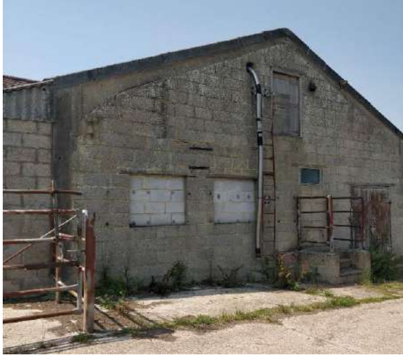
Photo 12: Northern elevation of B11.
