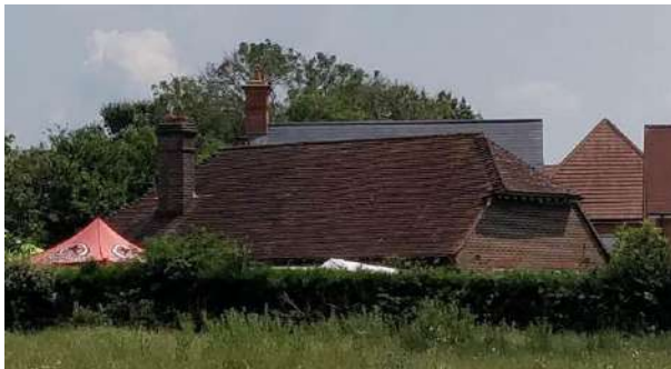
Photo 7: Western elevation of B7.
