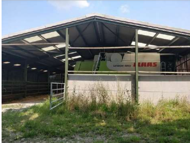
Photo 18: Southern elevation of eastern section of B15.
