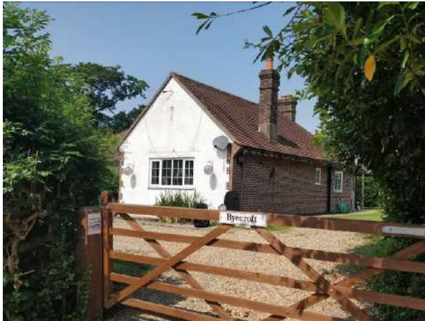
Photo 6: Northern and eastern elevations of B7.
