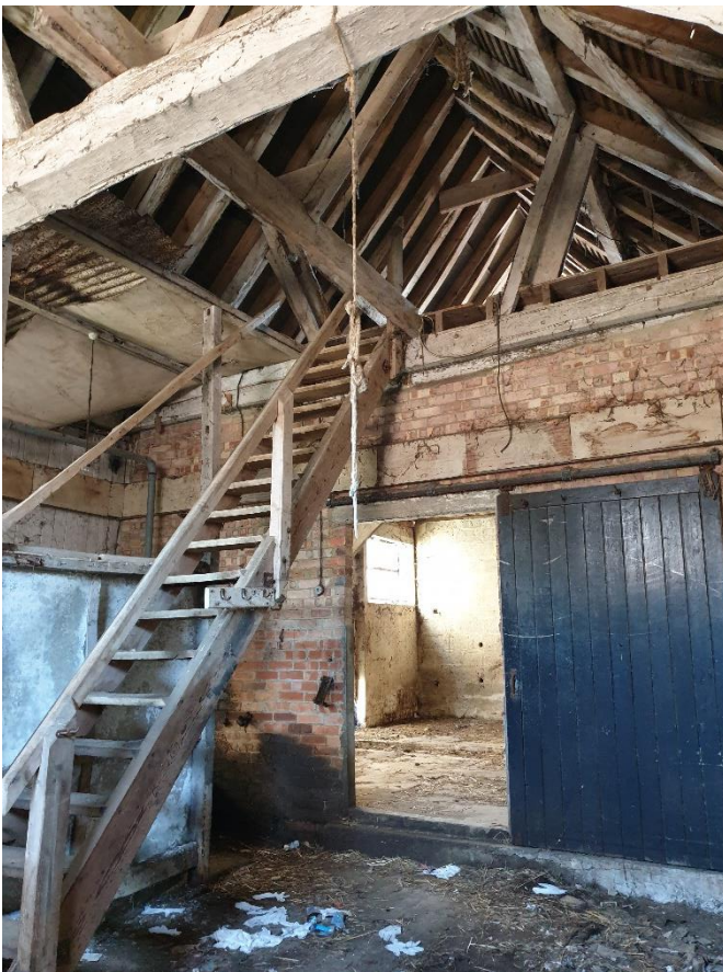
Figure 19: Interior of Barn A, showing timber frame with later alterations.
