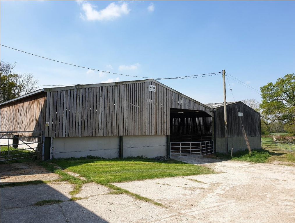
Figure 28: Barn H, early twenty-first century.
