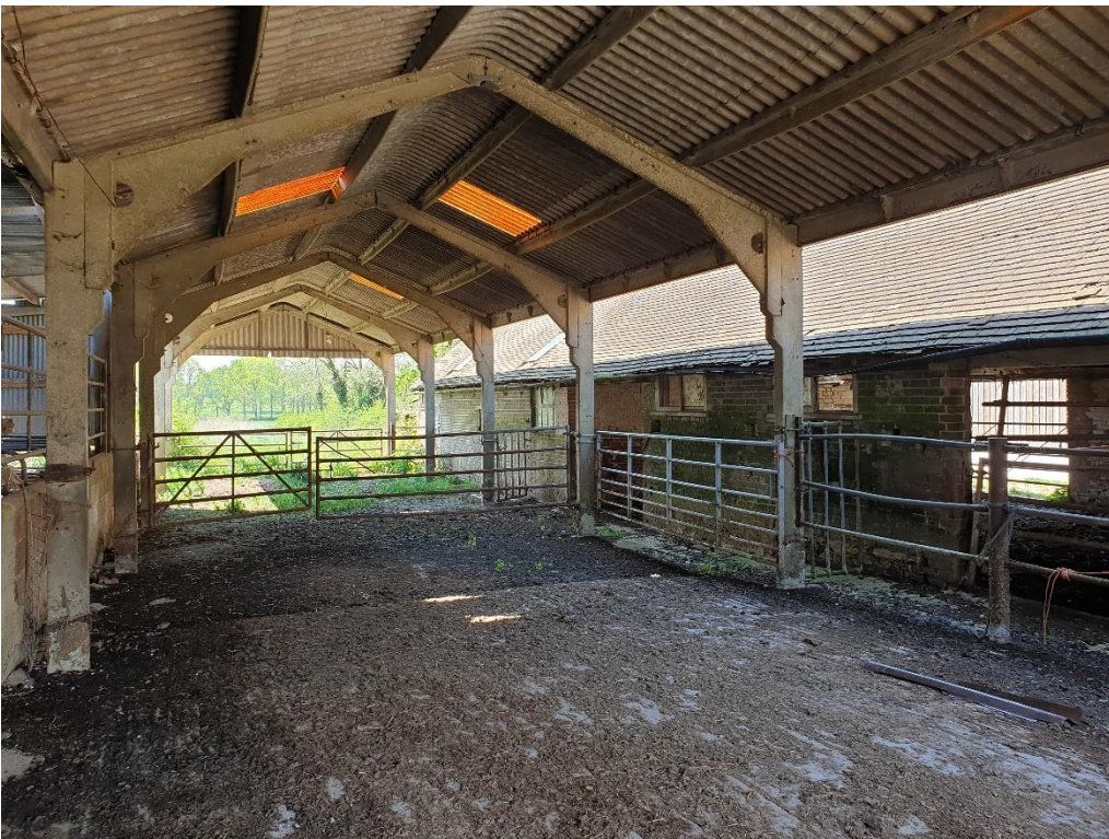
Figure 25: Barn E looking south, with concrete frame (Barn D to the right and Barn F to the left), late twentieth century.
