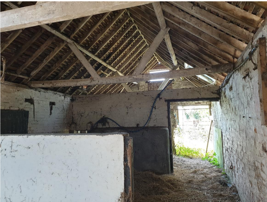
Figure 23: Interior of Barn C
