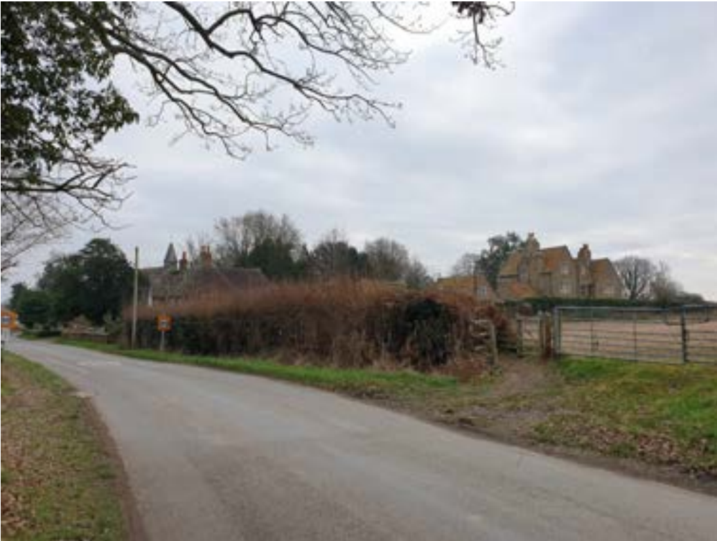
Figure 34: Southwater House, Grade II (right)
