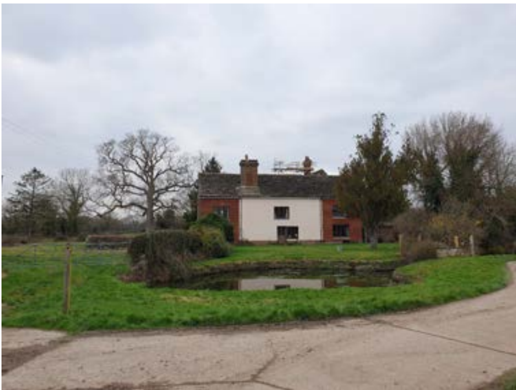
Figure 17: Great House Farmhouse, Grade II* in 2022. The Site is generally unchanged when visited in November 2025, although the scaffolding has been removed to the chimney.
