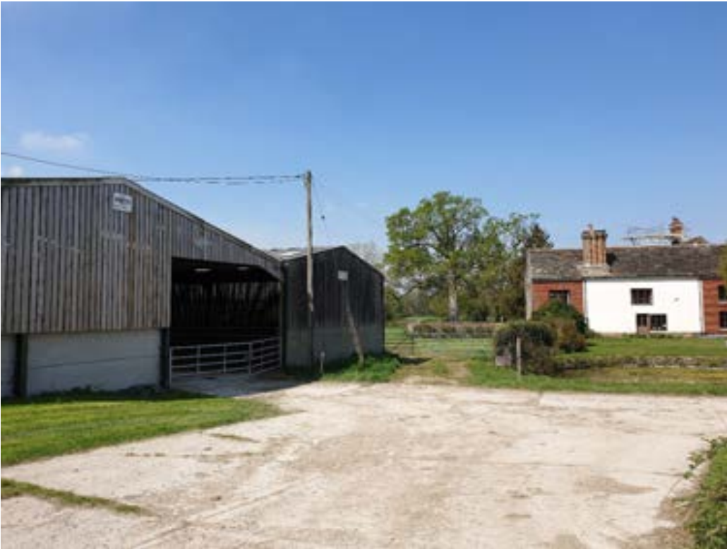
Figure 22: Barn H, which blocks views from the surrounding areas to the south towards Great House Farmhouse (2022).
