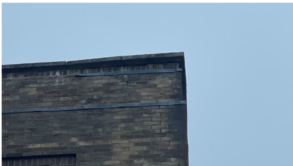
Plate B.6 Example of crumbling mortar below concrete eaves
