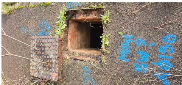
MH31X_ebb73134-f690-408e-8e0d-5e6dd5cd9f5c_20241125_104914.jpg, 00:01:07, 14.10 m Finish node, manhole, reference: MH41
