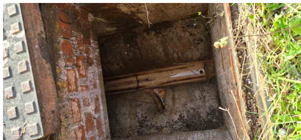
MH30X_a250596f-879c-4699-83ad-ff6263b89e11_20241125_104630.jpg, 00:00:01, 0.00 m Start node, manhole, reference: MH30
