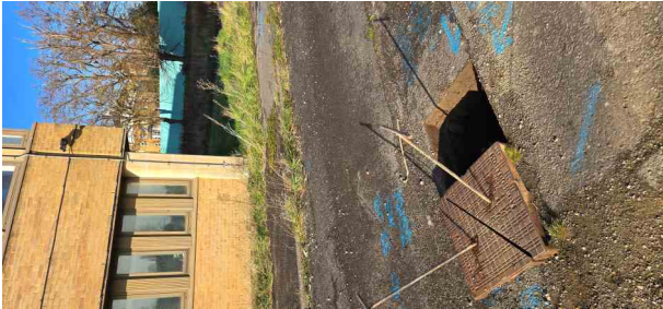
MH61X_e9efd8cd-0511-4080-8fd8-b2573383b329_20241125_135532.jpg, 00:00:01, 0.00 m Start node, manhole, reference: MH52
