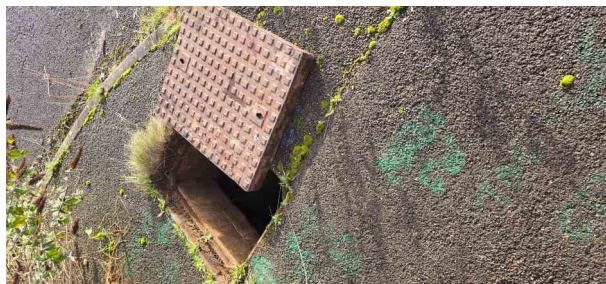
MH30X_36e63094-db5f-4636-ba2e-040563ca36ee_20241125_105029.jpg, 00:00:41, 6.18 m Finish node, manhole, reference: MH31
