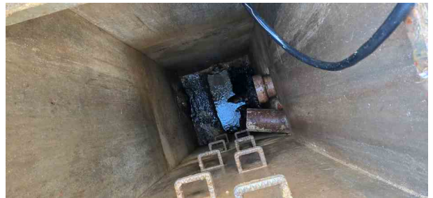
MH63X_fc3eee03-1a09-4fa9-a55e-c192e3ece00d_20241125_142804.jpg, 00:00:41, 7.64 m Finish node, manhole, reference: MH69
