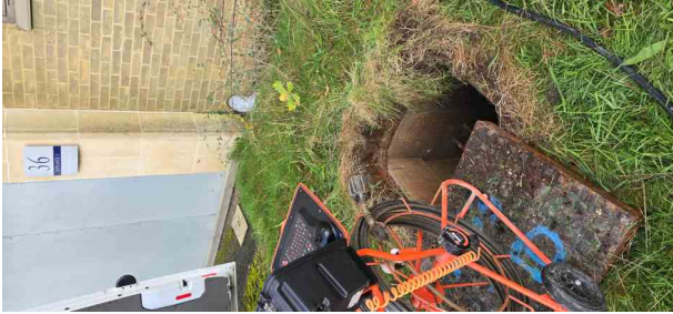
MH63X_84e43519-7d21-40aa-bcb9-b75b2af84fb4_20241125_142650.jpg, 00:00:01, 0.00 m Start node, manhole, reference: MH63
