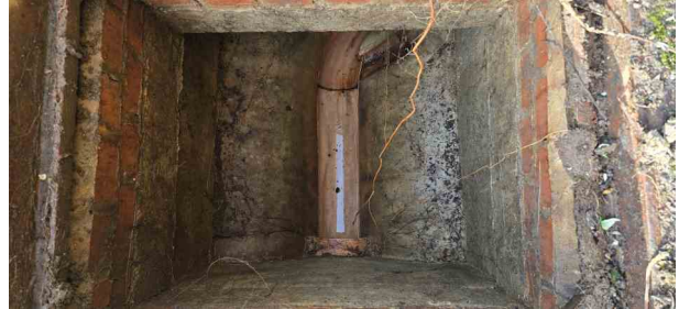
MH28X_122d1d2b-3703-4886-af15-0fd485a07d1e_20241125_104619.jpg, 00:00:01, 0.00 m Start node, manhole, reference: MH28
