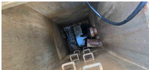
MH64X_b008573f-6747-4f00-aa6c-8ff2cf7564c6_20241125_142612.jpg, 00:00:50, 12.02 m Finish node, manhole, reference: MH69
