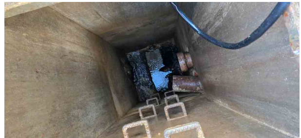
MH70X_482b3a68-3968-4f9b-934f-2755644c4826_20241125_142839.jpg, 00:00:26, 0.50 m Finish node, manhole, reference: MH69
