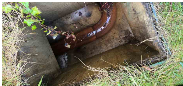
MH64X_d5373b3c-21a3-474c-b060-ec25bf1d1ca6_20241125_142625.jpg, 00:00:01, 0.00 m Start node, manhole, reference: MH64
