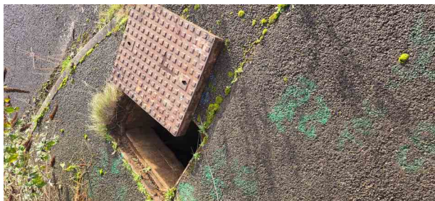
MH31X_1b539d62-dc46-4c8c-884b-19607f4dc15a_20241125_104636.jpg, 00:00:01, 0.00 m Start node, manhole, reference: MH31
