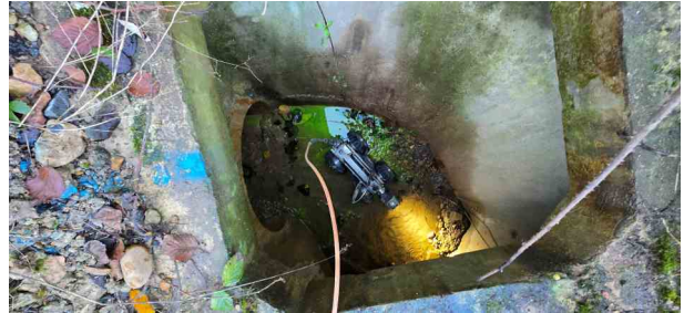
X_eef80fef-569a-412d-a87a-84c72ef6bb35_20241125_144828.jpg, 00:00:01, 0.00 m Start node, manhole, reference: MH92
