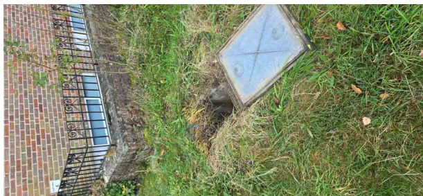
MH66X_af767249-9a80-4ee8-a502-89d04811b755_20241125_143053.jpg, 00:00:01, 0.00 m Start node, manhole, reference: MH66
