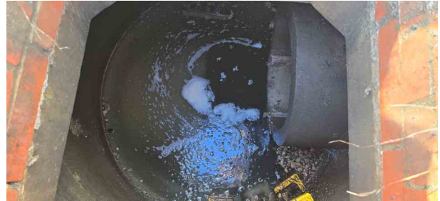
MH50X_3d1301d5-ca3e-409b-a436-1ac2832fe5e6_20241125_123435.jpg, 00:00:01, 0.00 m Start node, manhole, reference: MH50
