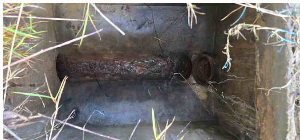
MH66X_2dc65504-d53d-443b-888b-a4185d0b8c0d_20241125_143058.jpg, 00:00:01, 0.00 m Start node, manhole, reference: MH66
