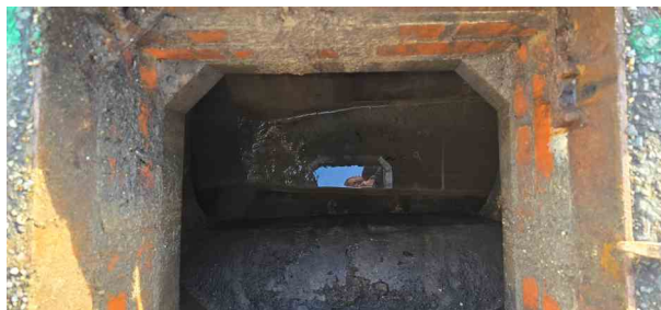
MH52X_db8eb618-e844-4224-9c42-6bb9f034aebd_20241125_115553.jpg, 00:00:01, 0.00 m Start node, manhole, reference: MH33
