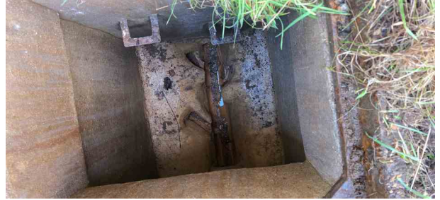
MH63X_f4076f48-0765-4e20-82e3-76d467fc6afd_20241125_142655.jpg, 00:00:01, 0.00 m Start node, manhole, reference: MH63
