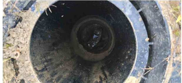
MH70X_16ffa554-662e-4a19-806b-834db8797b30_20241125_142815.jpg, 00:00:01, 0.00 m Start node, manhole, reference: MH70
