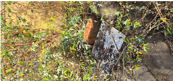
MH29X_70c4b88e-c05f-4202-9809-390d6086d4fd_20241125_113035.jpg, 00:00:47, 7.64 m Finish node, manhole, reference: MH27
