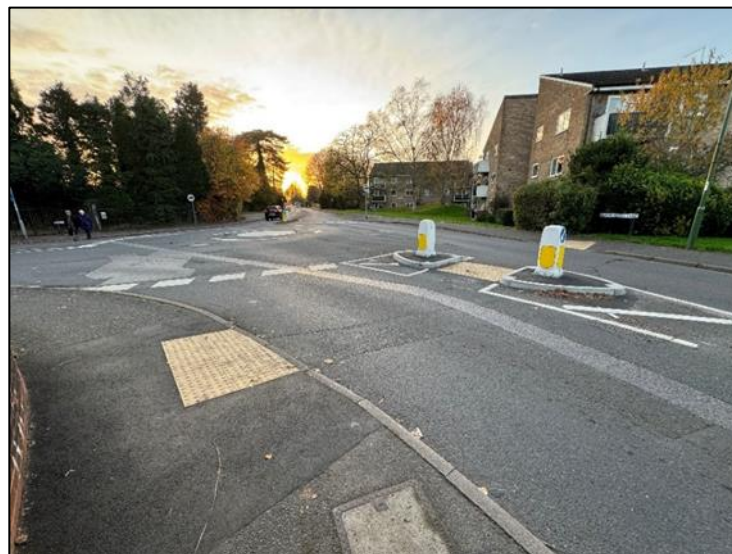
Photograph 4: Uncontrolled Crossing with Tactile Paving on North Heath Lane
