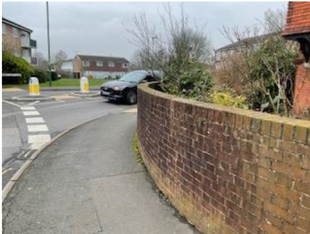
Figure 4: Wall restricting intervisibility at proposed crossing point.
