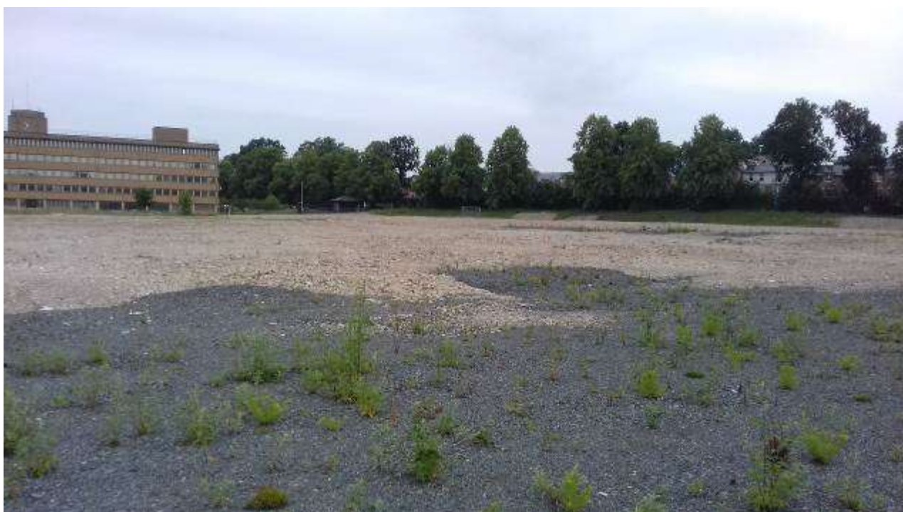
Photo 6 – Image showing areas of made ground rubble and road stone infill in areas which were excavated. Image looking north west across the site.
