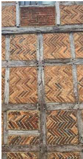
Herringbone brickwork
