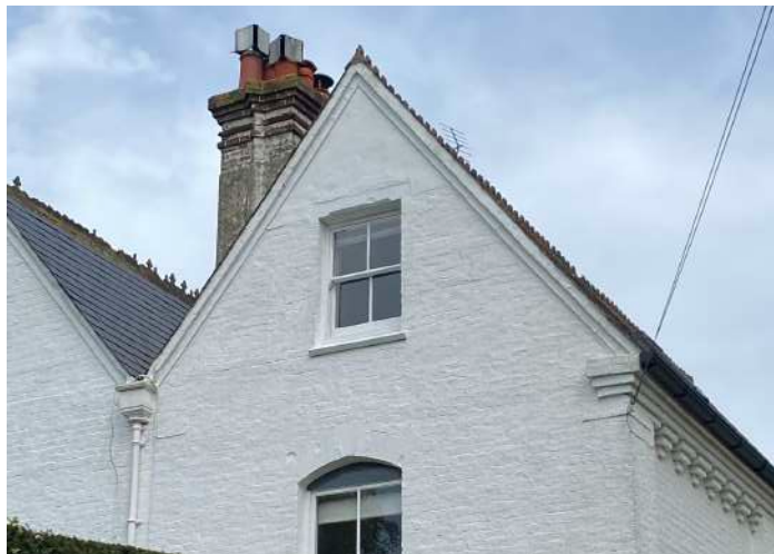
Brick detailing under eaves and roofline.
