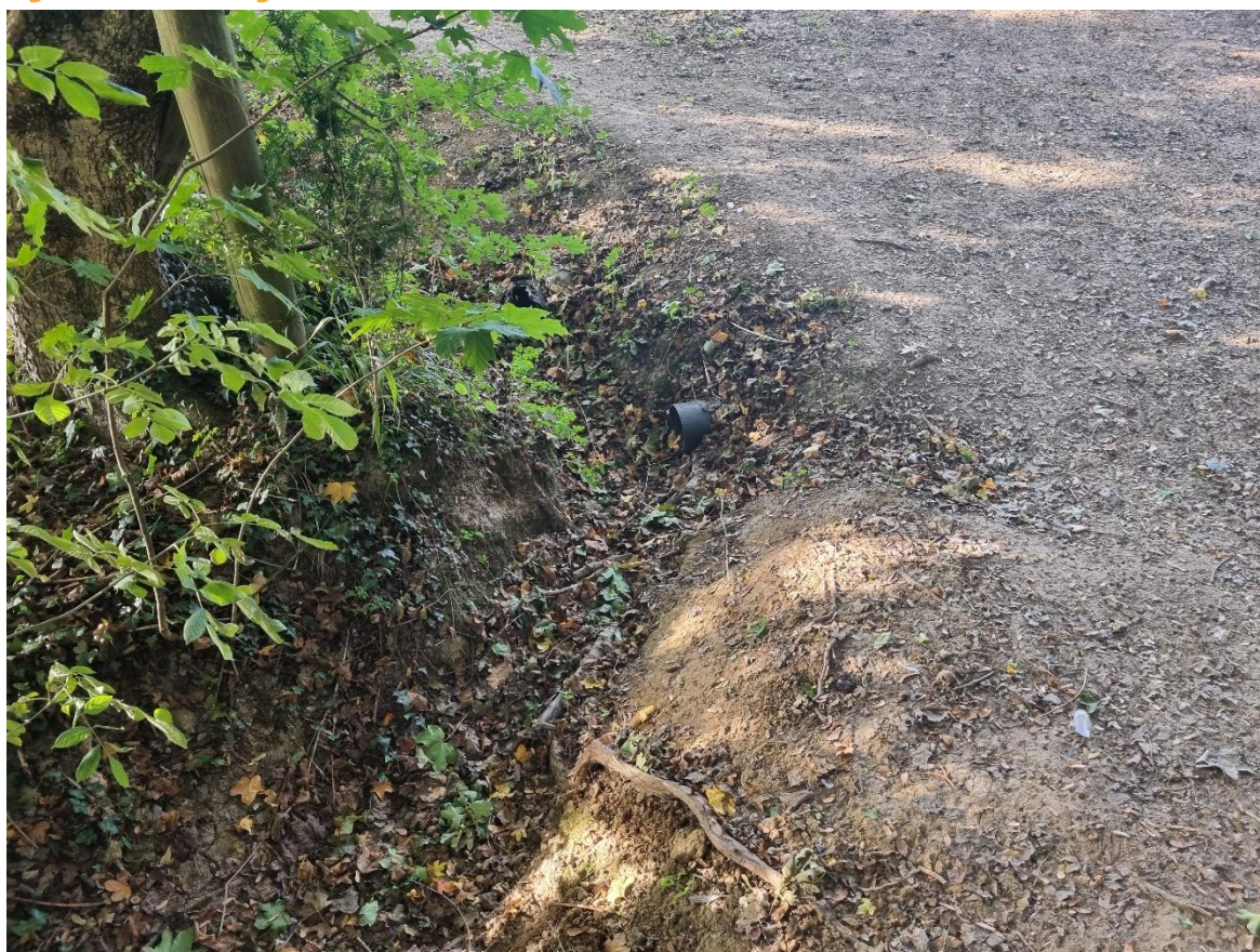
Figure 2.1 – Existing 100mm diameter outfall to the watercourse further downstream
