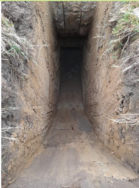
Plate 4 – Ground conditions encountered in TP1
