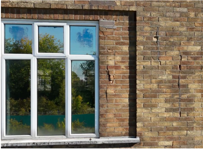
Fig 8 – cracking to external walls
