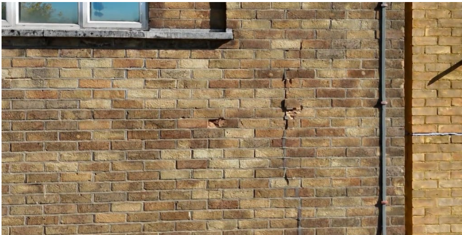
Fig 7 – evidence of corroded wall ties
