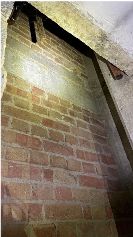
Plate B.7 Brickwork of lift shaft in basement level
