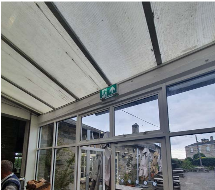
uPVC roofing to the clocktower cafe over historic timber frame
