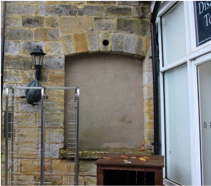
Existing blocked up historic window opening to be reinstated
