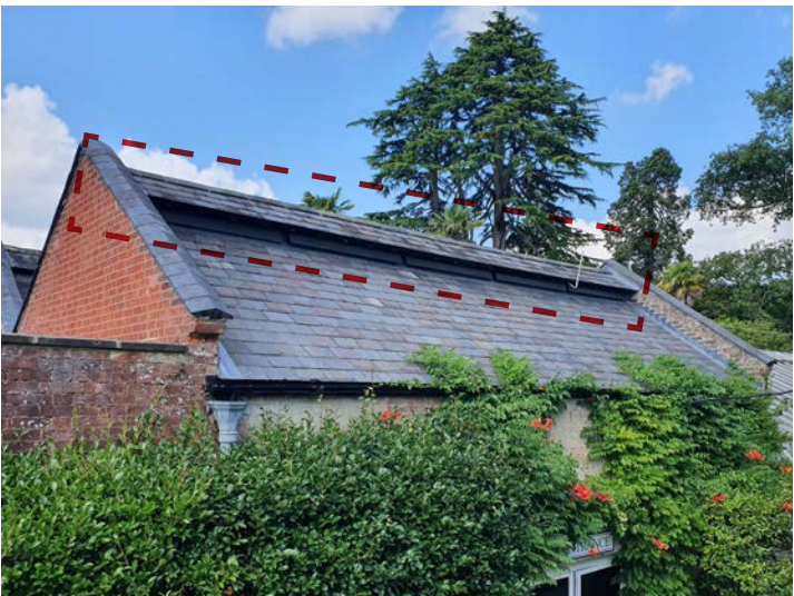
Existing historic ventilation detail to the pitched roof of the Former Generator Block
