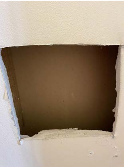
Opening up works identified a modern partition between Bedroom 1 and Bathroom
