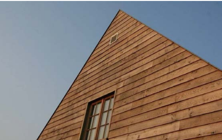
Weathered timber boarded wall - Image by SPP
