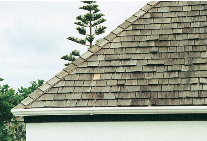
Weathered timber shingle roof example - image by Branz
