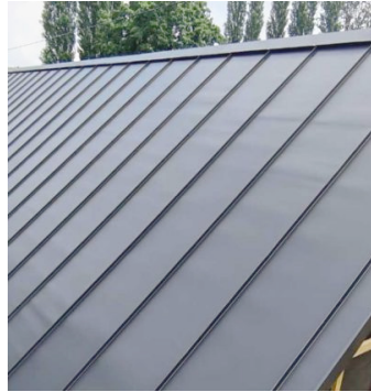
Metal standing seam roofing
