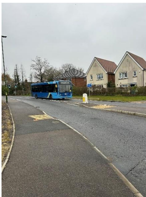
Photograph 3: Pedestrian Crossing on Mill Straight
