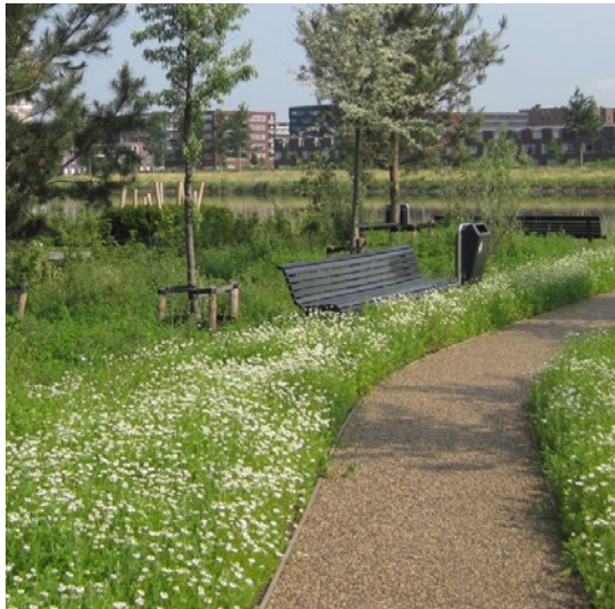
Self binding gravel footpaths through meadow
