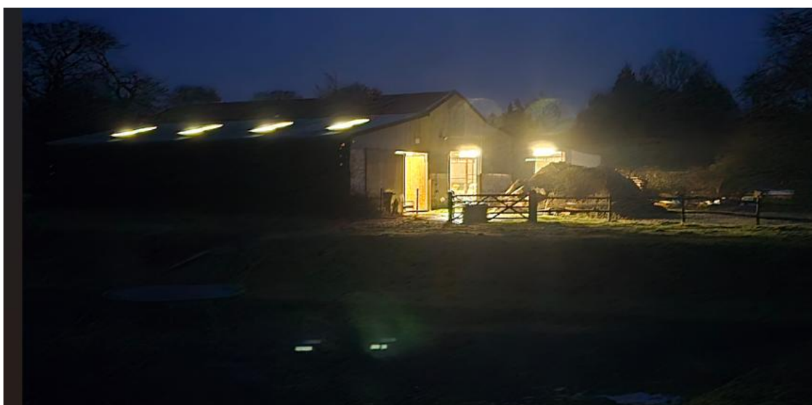
Figure 11- Former Barn sough to be Demolished
