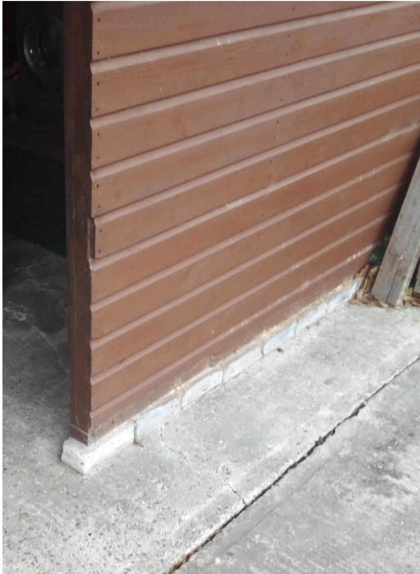
This photograph shows the base of the timber wall with a brick course onto a solid concrete slab. All in good condition
