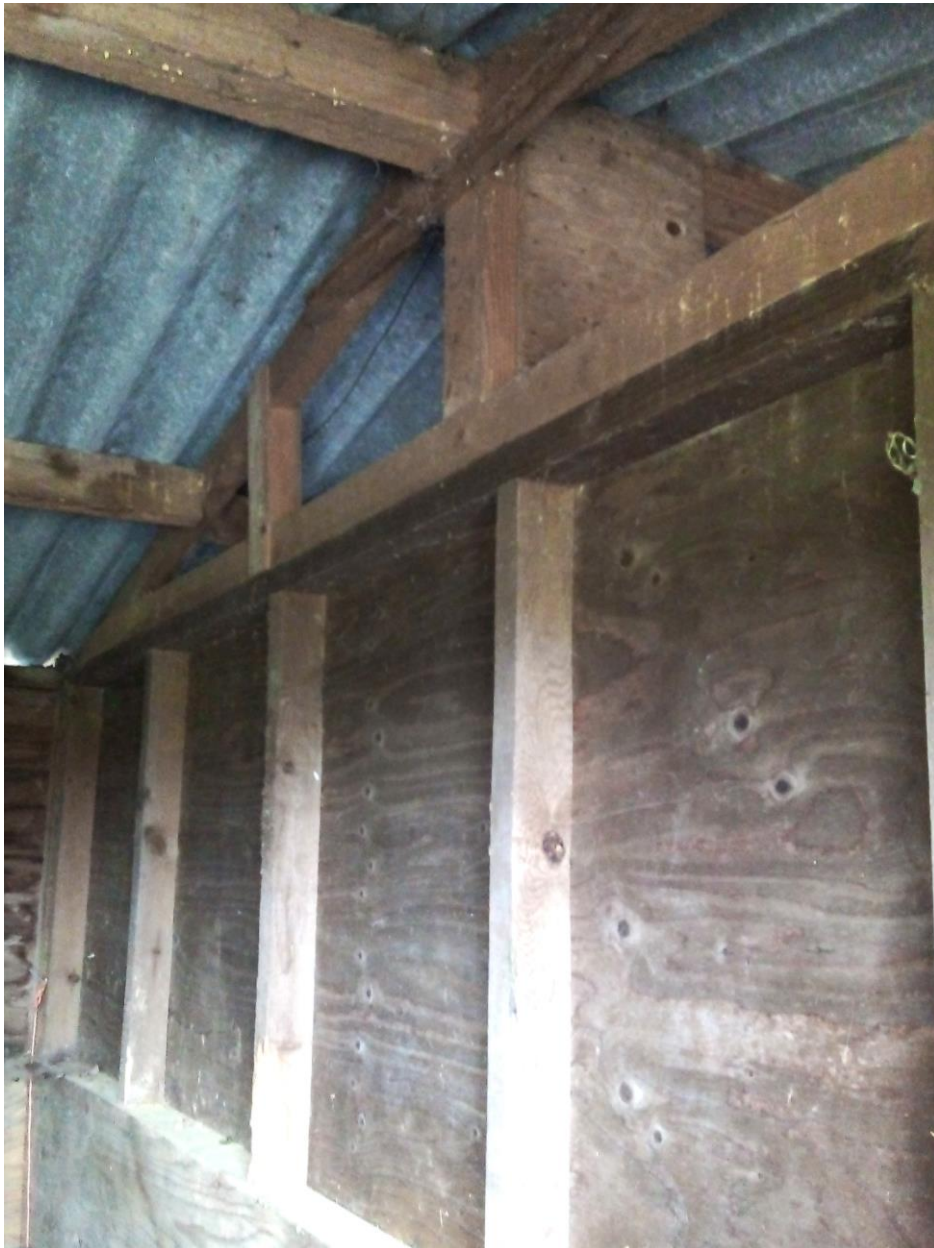
General internal view of roof structure - showing the internal partitions and purlins.
