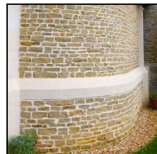
Stonework Detailing: Local Horsham or Fittleworth rubblestone in natural mortar. Complimentary recon. stone cill detailing where denoted.
