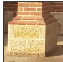
Columns: plinth bricks with stone bases.
