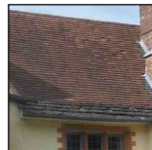
Roof sprocket: Horsham stone type sprocket detail
