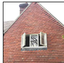
Vertical Tile-Hanging: Heritage Tiles - Clayhall Medium Blend clay plain tile.
