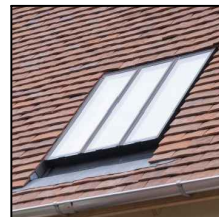
Rooflights: Black conservation type set with low profiles.
