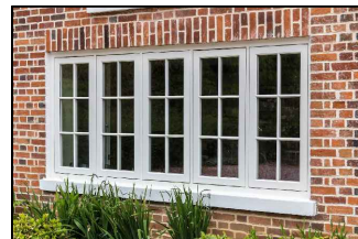
Windows and Doors: Painted timber framed, double glazed flush casement windows and doors with stone cill detailing.
