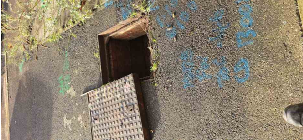
MH28X_e42b9812-bda0-4a33-aaa0-95b41106b23d_20241125_104542.jpg, 00:00:01, 0.00 m Start node, manhole, reference: MH28
