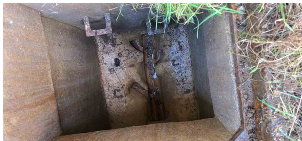
MH63X_f4076f48-0765-4e20-82e3-76d467fc6afd_20241125_142655.jpg, 00:00:01, 0.00 m Start node, manhole, reference: MH63
