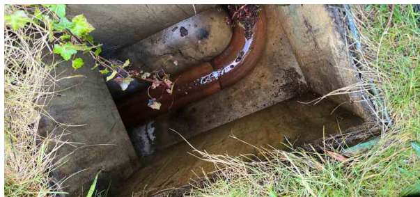
MH64X_d5373b3c-21a3-474c-b060-ec25bf1d1ca6_20241125_142625.jpg, 00:00:01, 0.00 m Start node, manhole, reference: MH64
