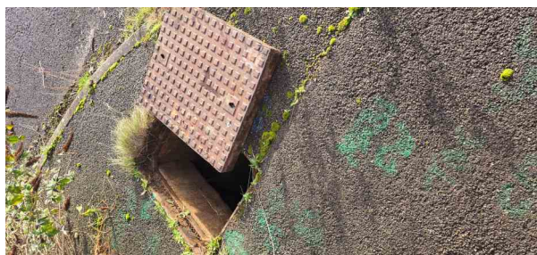
MH30X_36e63094-db5f-4636-ba2e-040563ca36ee_20241125_105029.jpg, 00:00:41, 6.18 m Finish node, manhole, reference: MH31
