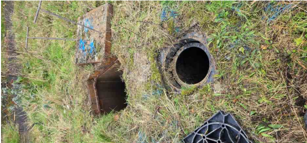
MH70X_952ce354-e7cf-4cab-a660-69bb7fe629e2_20241125_142811.jpg, 00:00:01, 0.00 m Start node, manhole, reference: MH70
