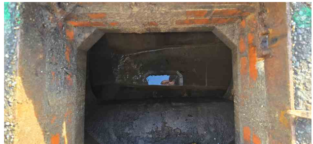
MH33X_115bf01f-265c-4dc9-b4e9-34a2b1cad7e3_20241125_145344.jpg, 00:03:02, 29.66 m Finish node, manhole, reference: MH33
