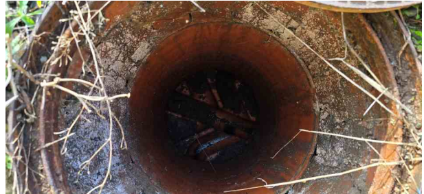
MH29X_900c1148-395f-4970-9e14-bc5ba8ed2804_20241125_113025.jpg, 00:00:01, 0.00 m Start node, manhole, reference: MH29
