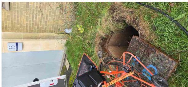
MH63X_84e43519-7d21-40aa-bcb9-b75b2af84fb4_20241125_142650.jpg, 00:00:01, 0.00 m Start node, manhole, reference: MH63
