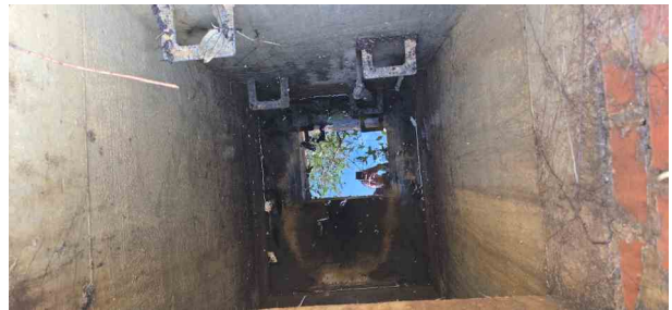
MH29X_d4099cf8-2af2-4cb6-8f57-635ec8cf874a_20241125_113040.jpg, 00:00:47, 7.64 m Finish node, manhole, reference: MH27
