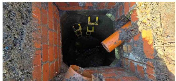
MH61X_95386cbb-045a-4908-ae61-5f8a9d181394_20241125_135443.jpg, 00:03:38, 32.41 m Finish node, manhole, reference: MH61
