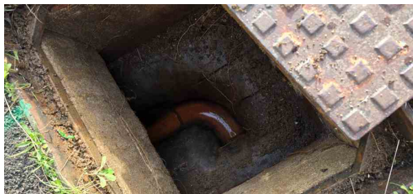
MH31X_692cda61-f981-4fc9-8050-62c47045bd7c_20241125_104641.jpg, 00:00:01, 0.00 m Start node, manhole, reference: MH31
