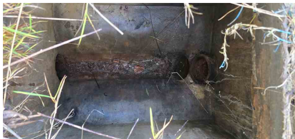
MH66X_2dc65504-d53d-443b-888b-a4185d0b8c0d_20241125_143058.jpg, 00:00:01, 0.00 m Start node, manhole, reference: MH66
