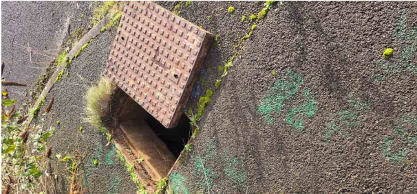
MH32X_84aef4aa-2e4e-4b57-8957-3d9b8e573ac4_20241125_105257.jpg, 00:00:01, 0.00 m Start node, manhole, reference: MH31
