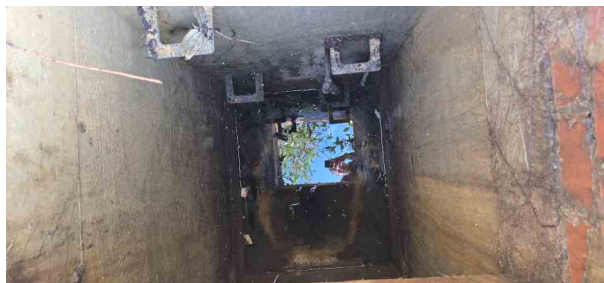
MH27X_fe3962d4-d31e-4d1b-9c03-24360ed70b05_20241125_113255.jpg, 00:00:01, 0.00 m Start node, manhole, reference: MH27
