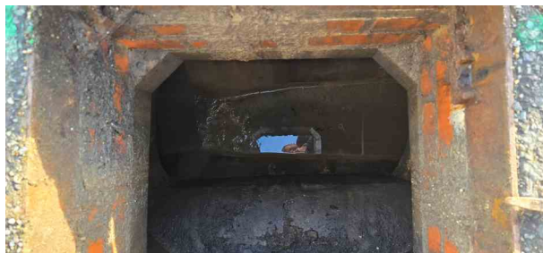
MH52X_db8eb618-e844-4224-9c42-6bb9f034aebd_20241125_115553.jpg, 00:00:01, 0.00 m Start node, manhole, reference: MH33
