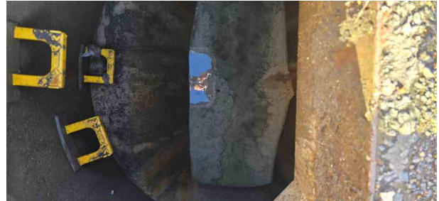
MH61X_449bec40-dc47-42f4-b402-821d3b46e9b5_20241125_135540.jpg, 00:00:01, 0.00 m Start node, manhole, reference: MH52
