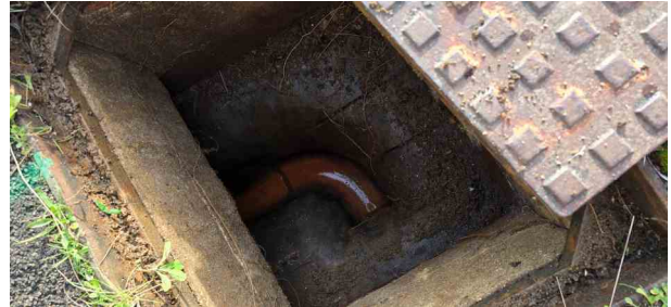
MH32X_9cfc2b80-a715-4459-88b9-deff1fcf4eab_20241125_105303.jpg, 00:00:01, 0.00 m Start node, manhole, reference: MH31
