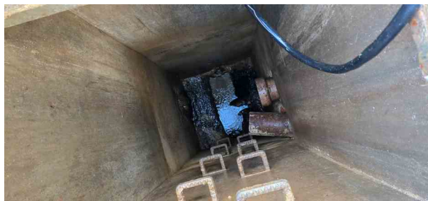
MH63X_fc3eee03-1a09-4fa9-a55e-c192e3ece00d_20241125_142804.jpg, 00:00:41, 7.64 m Finish node, manhole, reference: MH69
