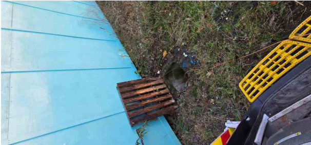
X_2586be45-4d85-47f3-9d48-08431449bb65_20241125_144824.jpg, 00:00:01, 0.00 m Start node, manhole, reference: MH92
