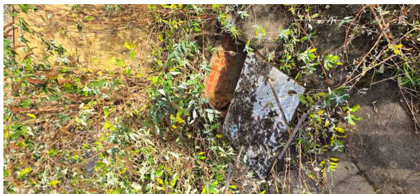
MH27X_576a0bc6-2da8-46f8-a3c9-27a2f49a2934_20241125_113251.jpg, 00:00:01, 0.00 m Start node, manhole, reference: MH27
