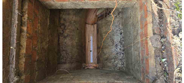
MH28X_122d1d2b-3703-4886-af15-0fd485a07d1e_20241125_104619.jpg, 00:00:01, 0.00 m Start node, manhole, reference: MH28
