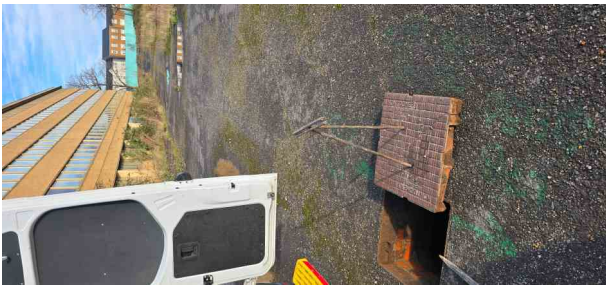
MH33X_2ca10918-82b4-4f2f-bf51-7afa06732a2f_20241125_145333.jpg, 00:03:02, 29.66 m Finish node, manhole, reference: MH33
