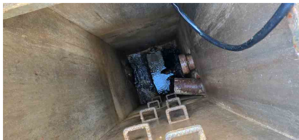
MH64X_b008573f-6747-4f00-aa6c-8ff2cf7564c6_20241125_142612.jpg, 00:00:50, 12.02 m Finish node, manhole, reference: MH69
