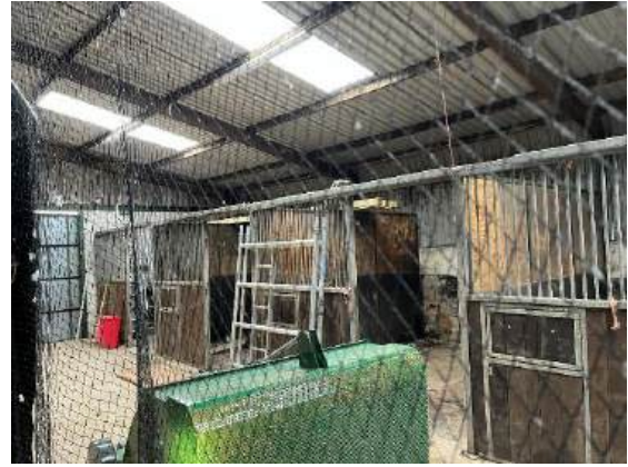
Photograph 8. Barn interior (western side)
