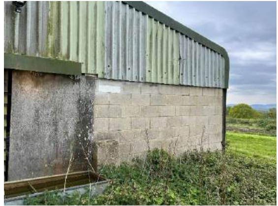
Photograph 4. North-western corner of on-site barn.
