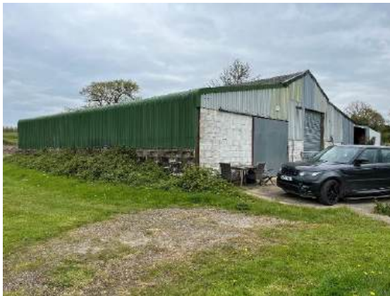
Photograph 9. South-western elevation of on-site barn.
