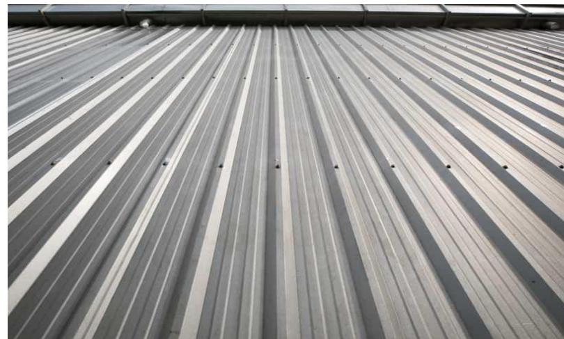
Grey Profiled Roof Sheet
